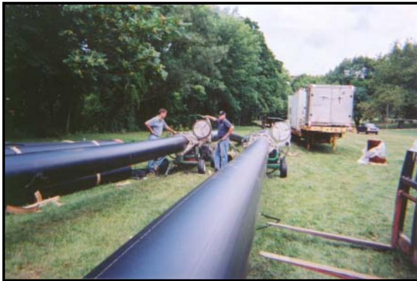
Thompson Pump crews operated two of six fusing machines around the clock in order to fuse the 12,800-feet of 18" HDPE pipe.
