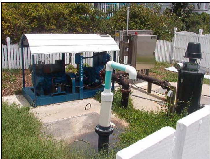
More of the permanent Thompson Pump emergency back-up pumps used by Regional Utilities in Walton County, Florida. The pumps automatically started when power was lost during the 2004 Florida hurricane season.
