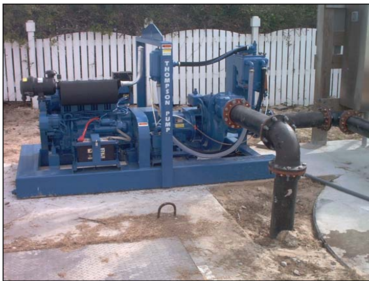
More of the permanent Thompson Pump emergency back-up pumps used by Regional Utilities in Walton County, Florida. The pumps automatically started when power was lost during the 2004 Florida hurricane season.
