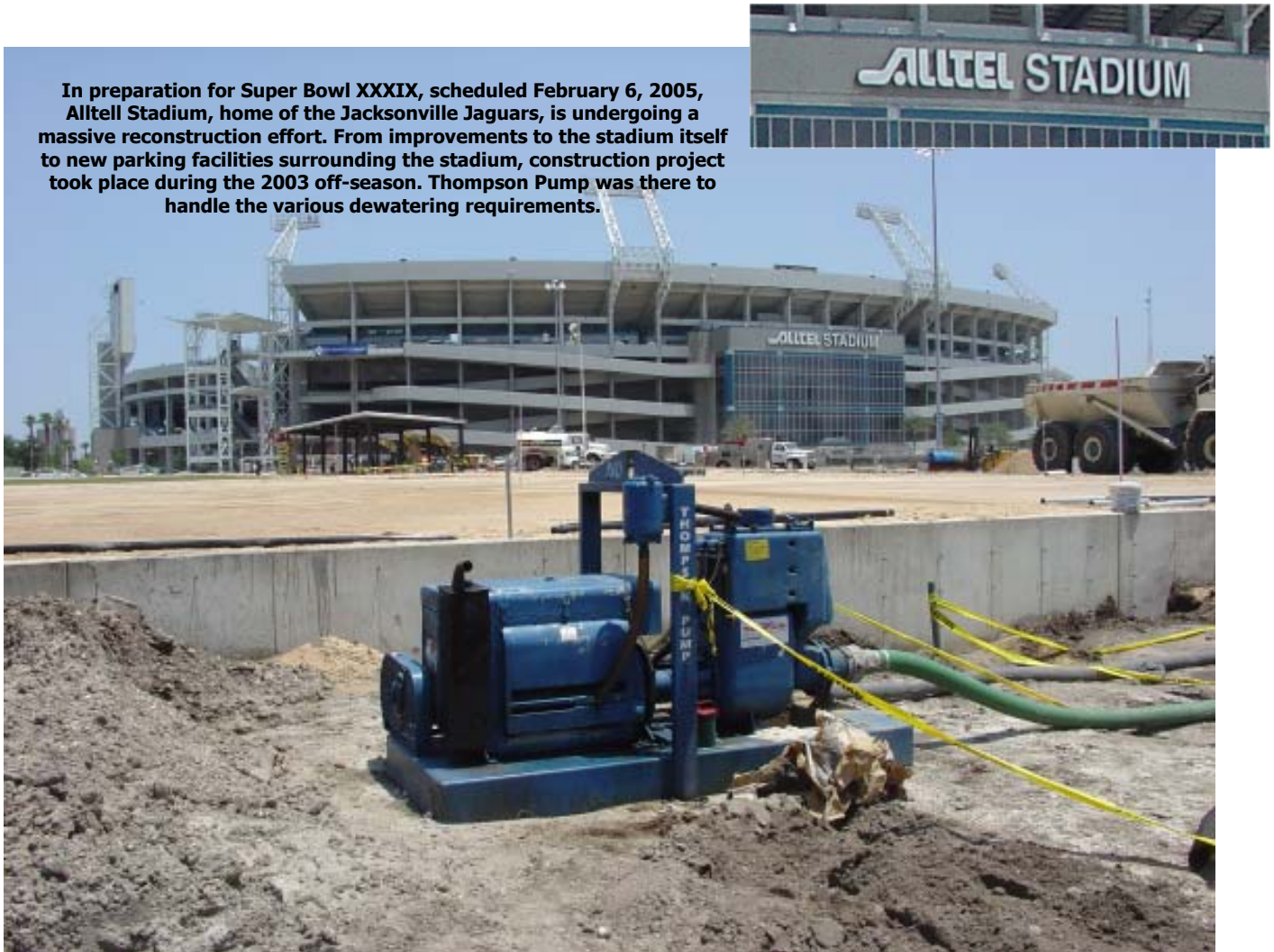
A Thompson Vacuum-Assisted Trash Pump does some dewatering in front of the stadium.
