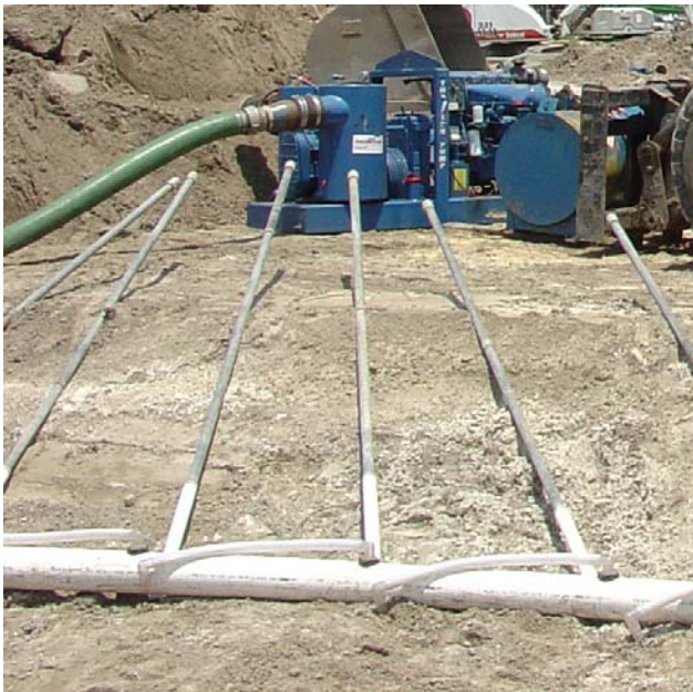
Above and Below: A Thompson Rotary Wellpoint Pump finished removing the groundwater to allow for construction, while work continues on the escalator system leading to the upper levels of the stadium.
