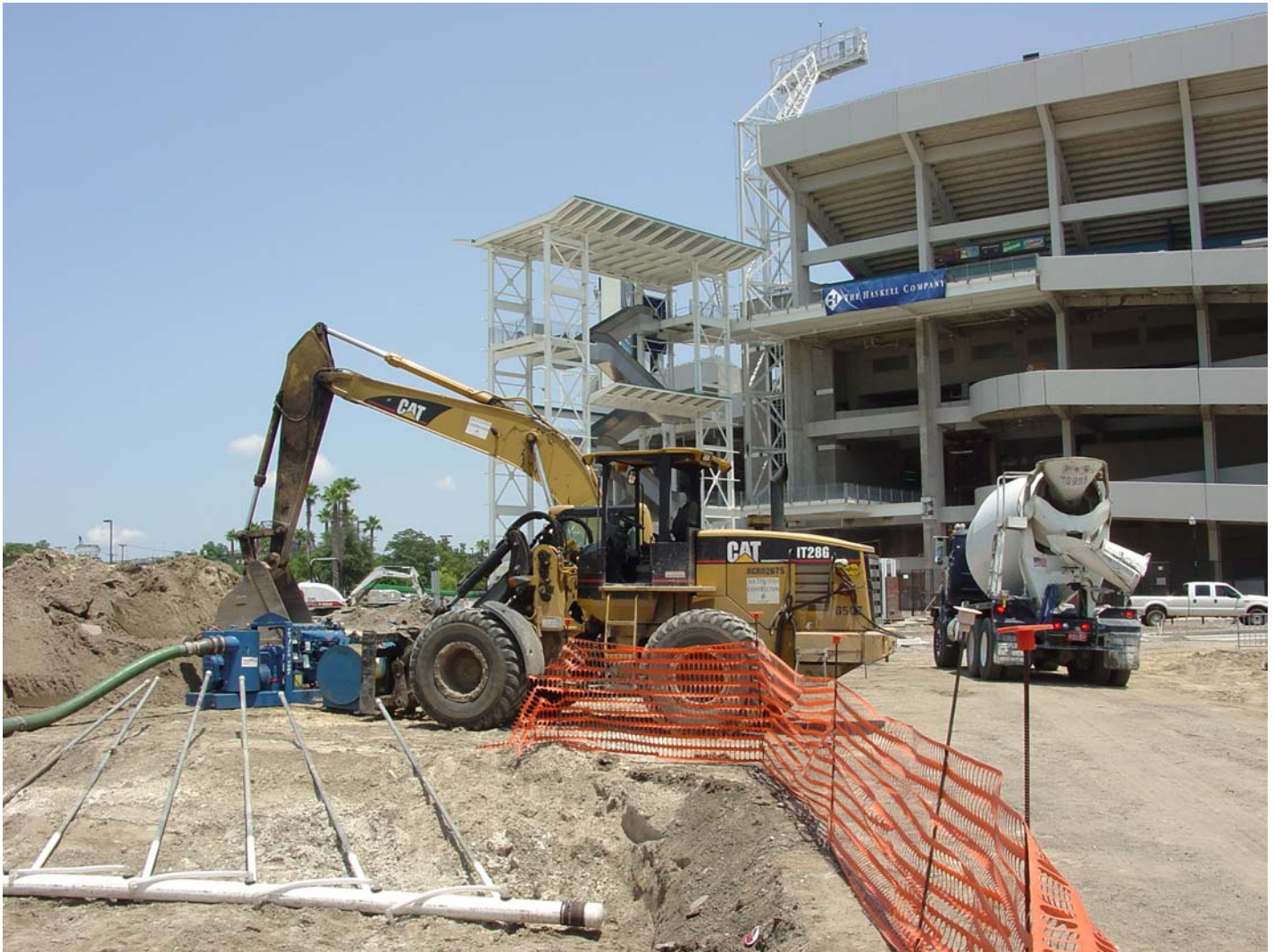
Above and Below: A Thompson Rotary Wellpoint Pump finished removing the groundwater to allow for construction, while work continues on the escalator system leading to the upper levels of the stadium.
