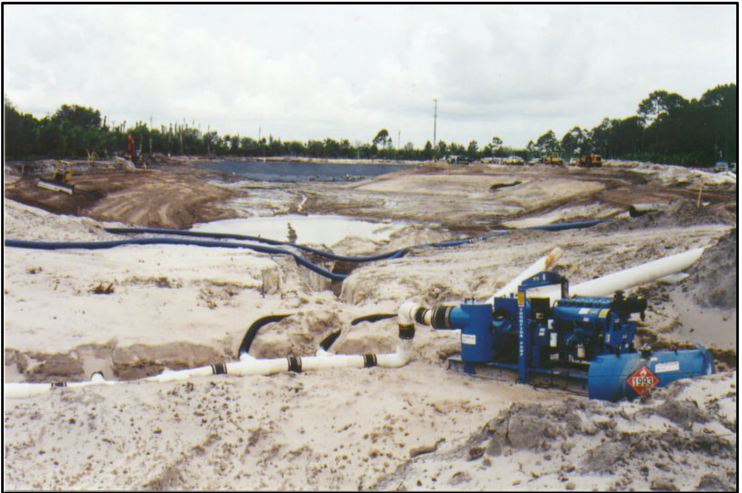
A Thompson Rotary Pump dewateres a section of the lake using sock while the rubber liner is being installed in the far section of the lake.
