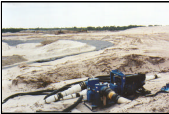
A Thompson Rotary Pump dewateres a section of the lake using sock while the rubber liner is being installed in the far section of the lake.
