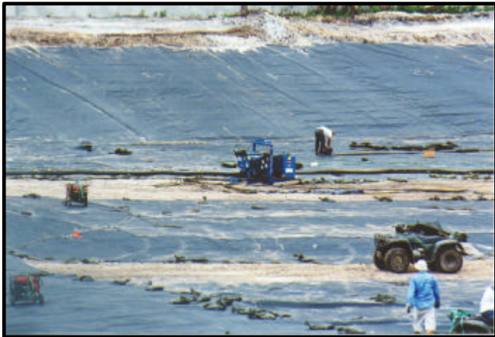
Above Left: A Thompson Hydraulic Power Unit is situated in the middle of lined area in order to remove unexpected rainwater using a Hydraulic Submersible Pump from a storm that hit in the middle of the project.
