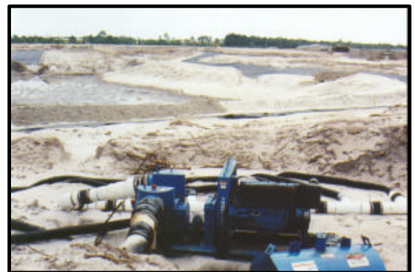
A Thompson Rotary Pump dewateres a section of the lake using sock while the rubber liner is being installed in the far section of the lake.
